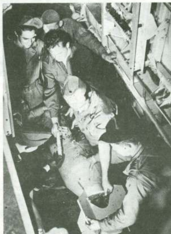
A series of bomb pictures by Arthur Mack, 367th pilot, shows the (1) bomb dump, featuring 500 pounders, (2) trailers of 1000 pounders arriving at the plane and having their tail fins mounted, (3) crew pushing the big bomb under the bomb bay, and (4) check details just before hoisting the bomb up to the shackle hanging on the right rack.
